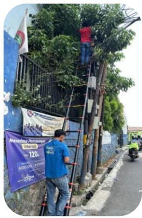
Installation of Wireless Access Points
